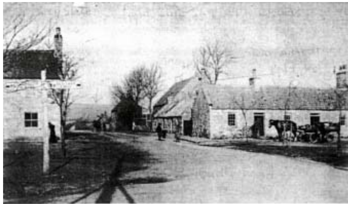
Old View Of Congregational Church on West Street (Windhill Street) See large house on the right after single storey cottage, with Manse beyond.
